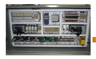
Electrical Control System with Ethernet Communication interface based in NI Compact RIO PAC Device
